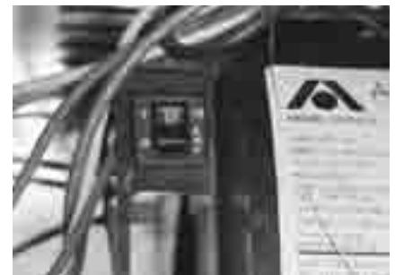
Furnace breaker – exterior location.
