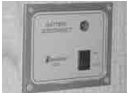
Battery Disconnect Panel Class C
