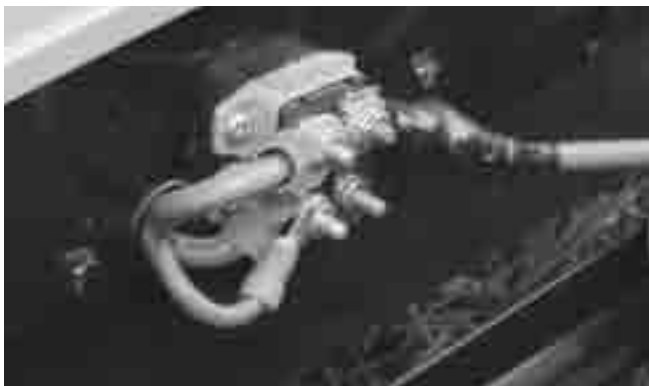
Travel Trailer 12V mini-breakers. (Front frame)
