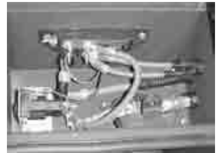
Gas Chassis / Mini-Home Class C battery disconnect solenoid and 12V mini-breakers
