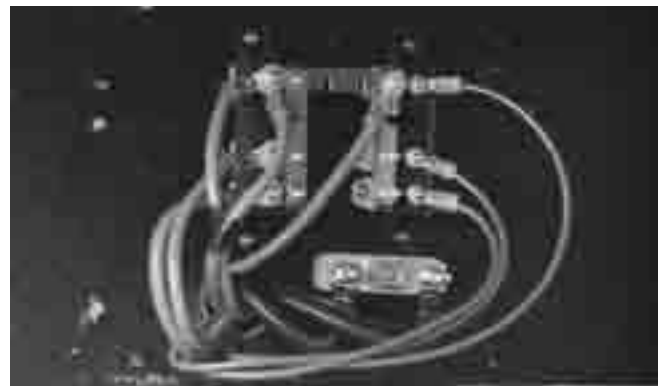
Fifth Wheel 12V mini-breakers. (Front compartment)
