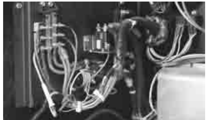
Rear Diesel battery disconnect solenoid and 12V mini-breakers. (Rear compartment)
