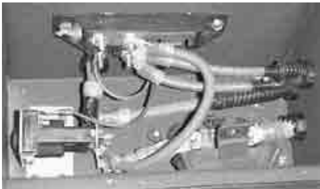
Mini-Home Class C 12V mini-breakers. (Under step area)
