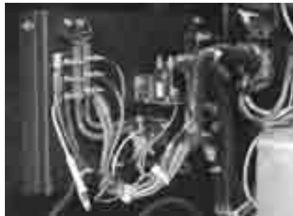
Rear Diesel battery disconnect solenoid and 12V mini-breakers
